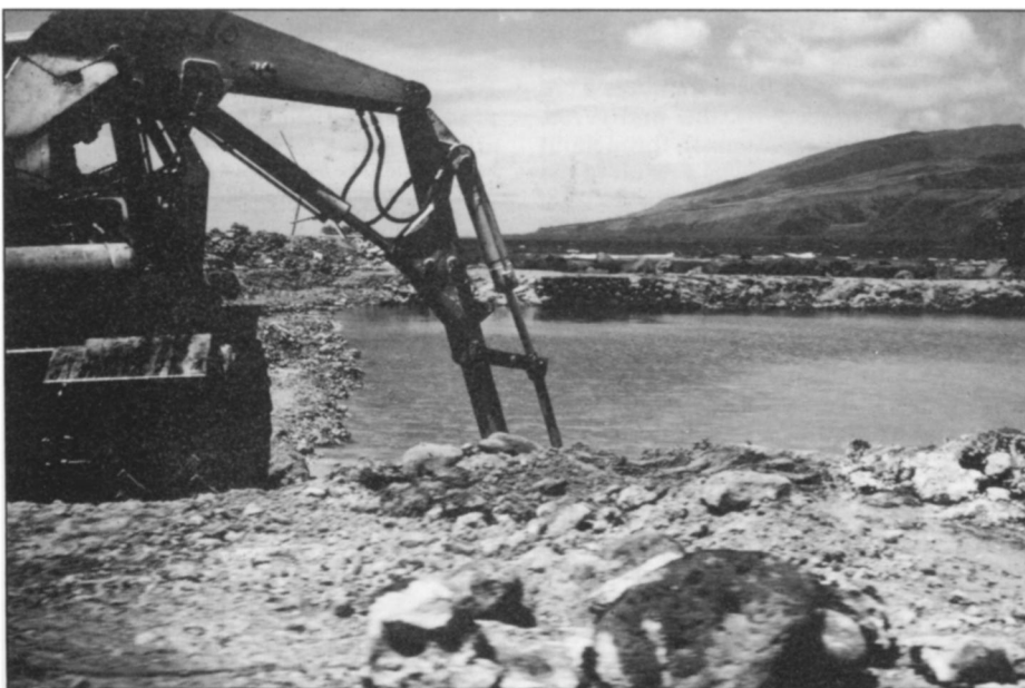
Dredging construction material from a lagoon on Tahiti (French Polynesia) pollutes adjacent waters and reduces the productive area of marine habitat. This is a problem that affects wide areas of the South Pacific. Photo: A Dahl.
